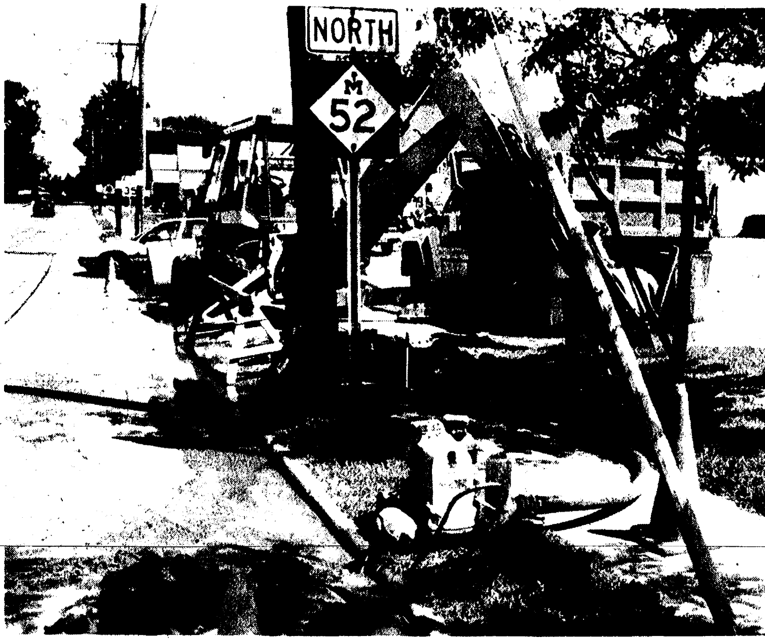
A WATER LINE BREAK between Chelsea Industries, Inc. and Tower Mart on Main St. kept village crews busy to contend with, such as a gas line in the area, as well as sand that continually caved in.
